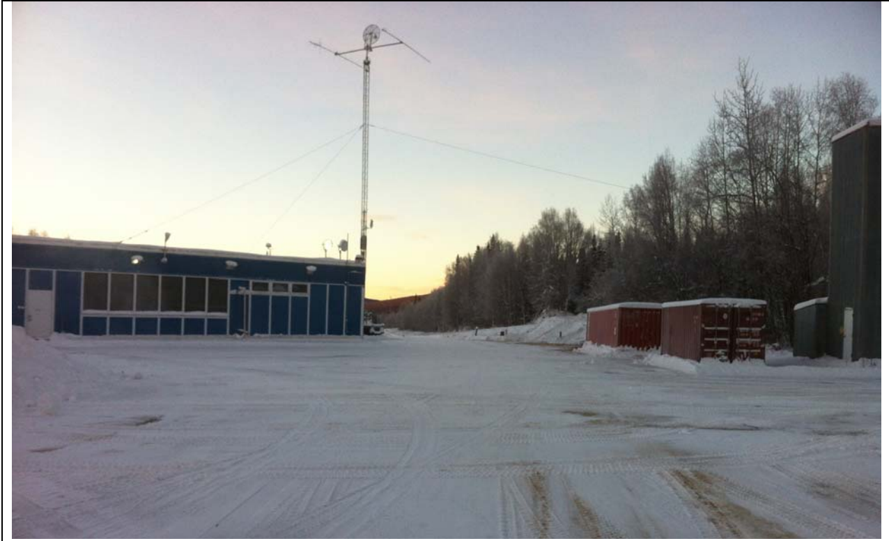
West View from VLBI Parking Lot
