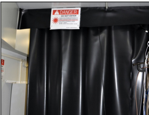
Figure 3-7: Beam blocking curtain inside the shelter
